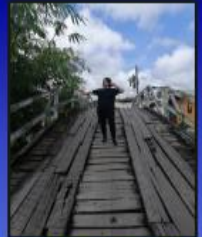
Old Wooden Bridge
